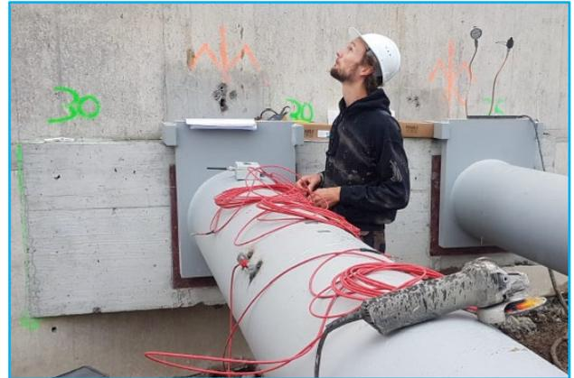
After welding the sensor end blocks, using a welding gauge, the sensor is installed, adjusted and the are cables connected to the wireless data logger located at the edge of the excavation pit. From the strain differences (reference to subsequent measurements) of the 3 strain measuring points, the forces are determined, based on the stiffness of the respective strut.
